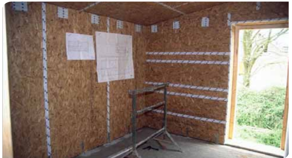
Figure 8 OSB-3 with joints taped
