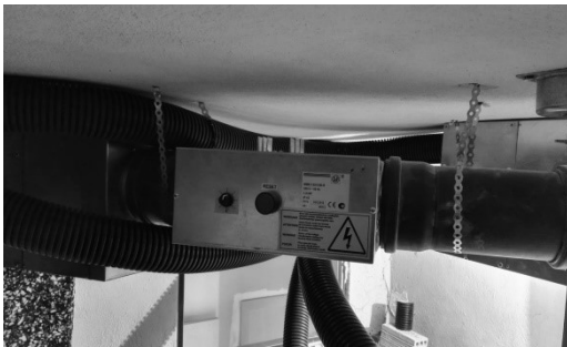
Figure 4: The after-heater
