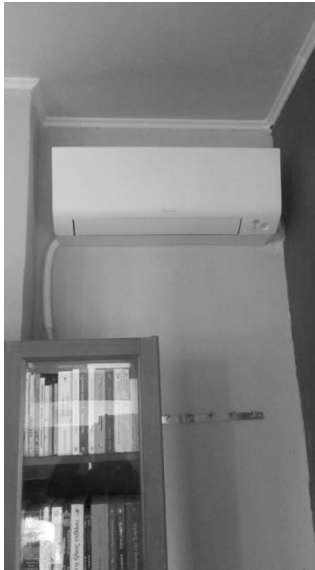
Figure 8: The installed Minisplit
