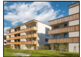
Socially compatible and highly energy efficient: apartment blocks built to the Passive House standard. © Neue Heimat Tirol
