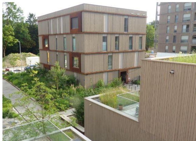
The Passive House district consists of eight buildings and includes ancillary facilities such as a communal kitchen. © Passive House Institute
