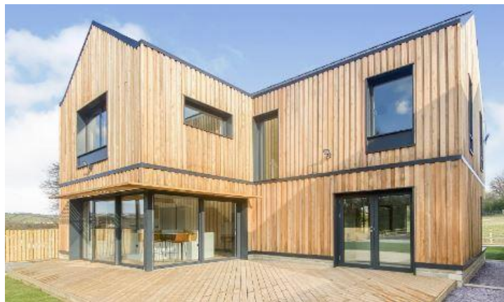
This Passive House building in Bradford, UK, can also be visited in person, ID 6447.
