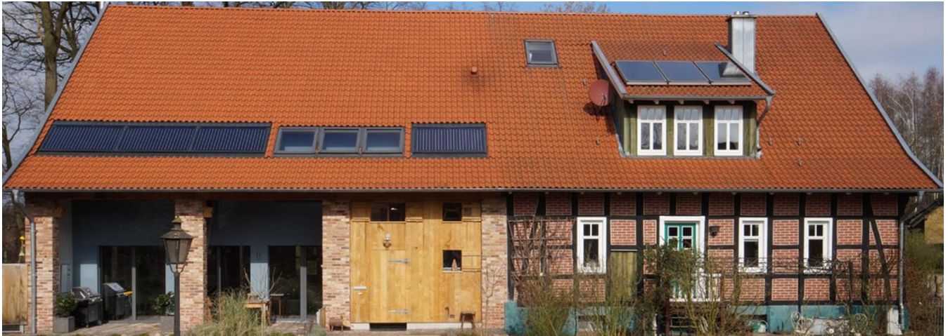
New within old: In North Rhine Westphalia's Steinhagen, the builders integrated their Passive House (I.) into a 100-year-old carriage house. The German public television channel ZDF was also impressed by the project and reports about it in the "Morgenmagazin". You can find the report by clicking on this link , it starts at 25:20. © Thomas Spooren
