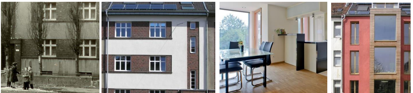
This row house in Mönchengladbach, also a city in the state of North Rhine Westphalia, is one of 12 identical building projects and has been retrofitted to the EnerPHit standard. The EnerPHit standard promises energy efficiency for existing buildings that comes close to the Passive House standard. The garden façade (r), too, profited from the retrofit. © bau grün!
