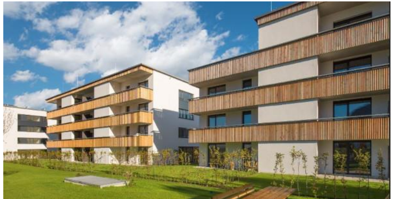
Energy efficient and cost-effective: social housing built by the housing group Neue Heimat Tirol in Kufstein, Austria. © Neue Heimat Tirol
