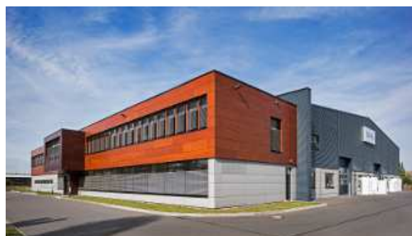
A Passive House in German Reinsdorf which is also the headquarters of a manufacturer of Passive House components.
