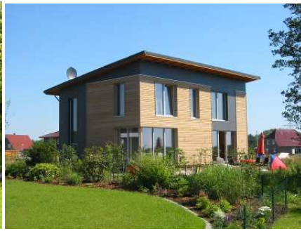
A single family home built to Passive House Standard in Westerstede/ Germany. Photo: Christian Gauler
